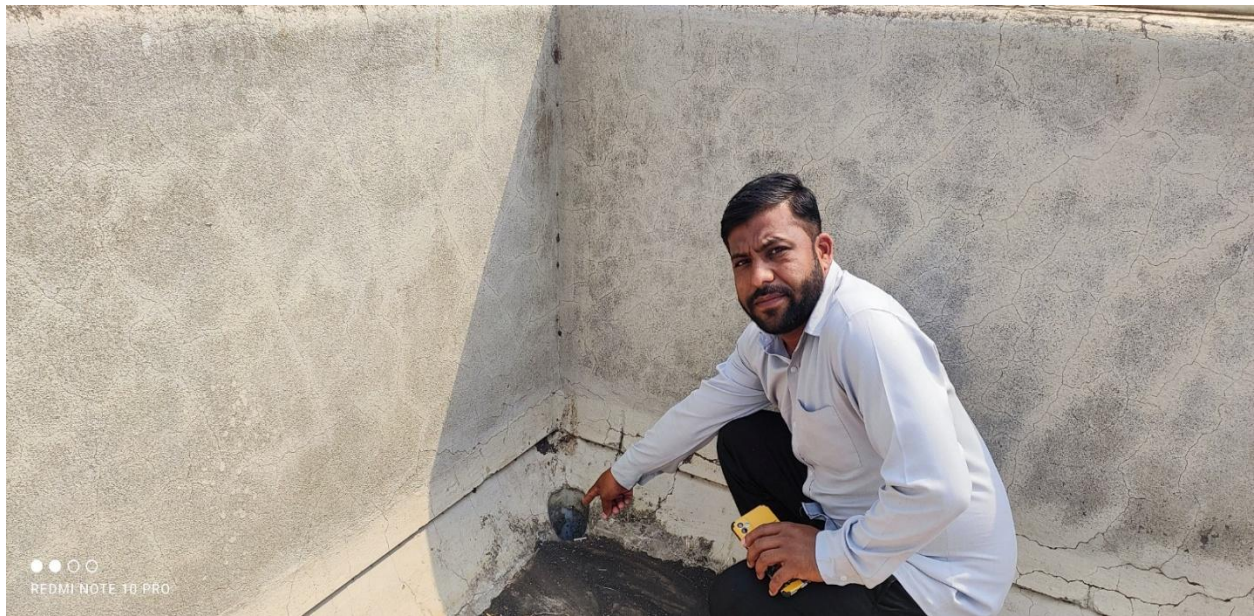
Fig 5.1: RWH inlets from terrace
